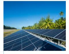
Solar energy, produced by 4,000 photovoltaic panels located along the runway, covers 75% of the resort's energy needs. These panels demonstrate how productive an unused space can be. Solar water heaters, meanwhile, satisfy almost all hot water needs from the hotel.
