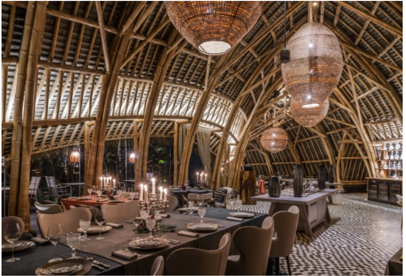
The restaurant at Sundy Praia, built of bamboo and palm fronds
